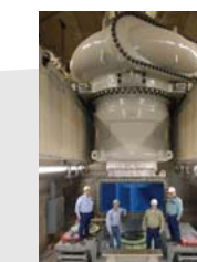
2011 Large scale centrifugal pump with world's highest efficiency level, supplied to Edmonston pumping station, USA.
