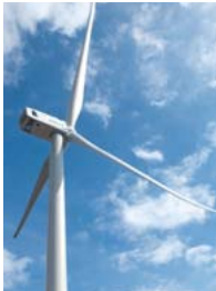
5.2MW wind turbine with downwind rotor
