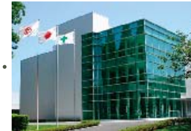
Mechanical Eng Lab. (Base for mechanical systems)
